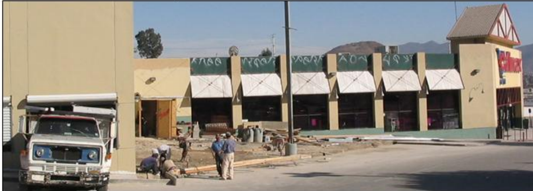
New location under construction in Tijuana, Mexico
