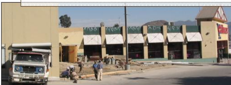
New location under construction in Tijuana, Mexico
